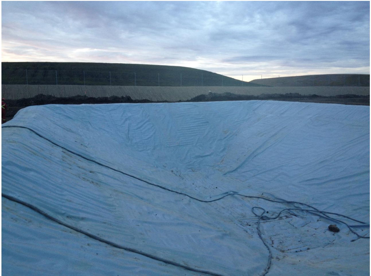
Figure 1: Completed Polyurea Pond
