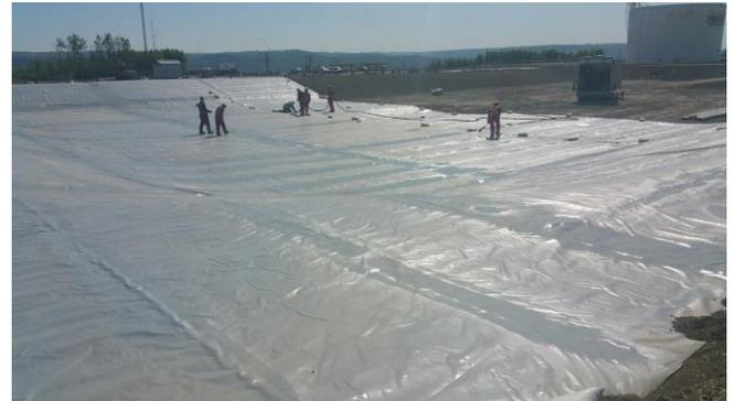
The 30'x30' panels were positioned in the containment area and joined using **PRECIDIUM™ ECS™ Fusion**. The panels showed very little shape memory from being rolled and laid flat when deployed. Installation began on the containment bottom, proceeded up the berms, and at the top of the berm were terminated in an anchor trench dug by the small backhoe.
