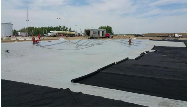
In total, the seven-member crew installed more than 60,000 square feet of **ECS™** and geotextile in just four days. QA/QC documentation was completed at each stage of the process to the satisfaction of the facility owner.
