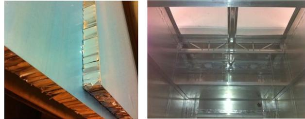
The Clean Room was a modular design using mill finish aluminum extrusions and panels. Basic wall panels consisted of two sheets of aluminum sandwiching and aluminum foil honeycomb. Walls were 2" thick; ceiling panels used the same design but are 1/2" thick. The ceiling consisted of a top plenum cap 10' high which provides the outer air seal and an 8' suspended inner ceiling holding the lights and HEPA filters.
