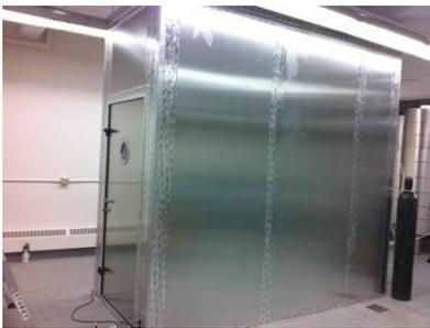
The outer 5'x10' airlock was built as the prototype room to test how well the clean room could be sealed.
