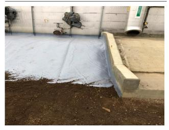
WEC's **PRECIDIUM™ ECS™** Tank Skirt was chosen by Suncor as the solution to minimize berm erosion and tank base corrosion. WEC's industry leading 15-year Warranty provides worry free maintenance for many years to come. For reference on this project or any other ECS™ installation, please contact WEC at the numbers below or visit us at <u>www.wecontain.com</u>.
