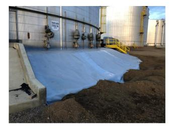
The entire 40 mil liner was pre-fabricated offsite utilizing WEC's industry-leading robotic application prespray system and was permanently fused together onsite with **PRECIDIUM™ ECS™ Fusion**.
